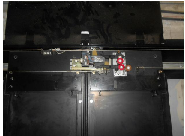
Photograph No. 4 – Landing door locks
