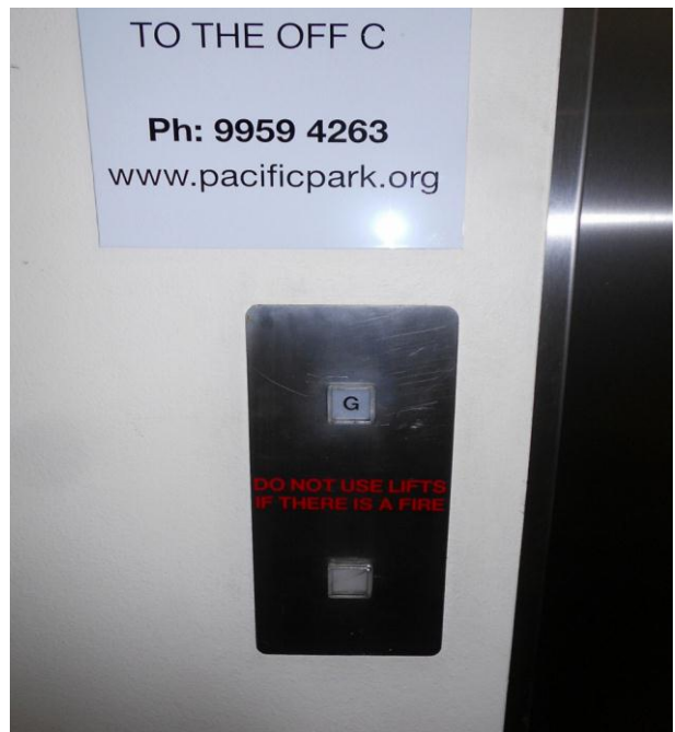
Photograph No.6 – Landing button panel
