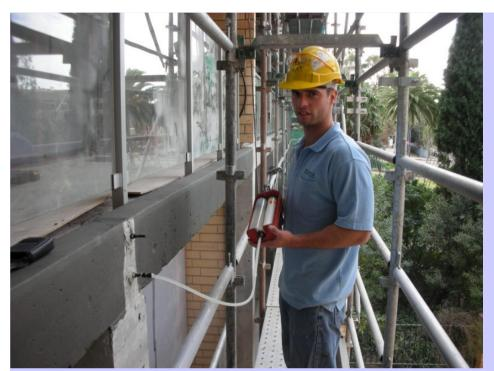
Following crack and spalling repairs the slab edges were coated with a modified cement based coating to reduce porosity and provide a suitable substrate for render application.
