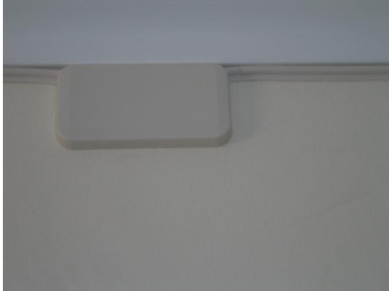
Proposed housing at unit door (with cabling)
